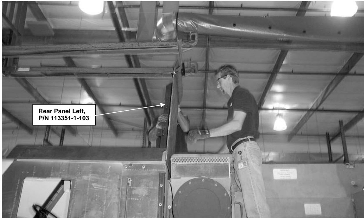
Figure 37. Rear Armor Panel installation.
